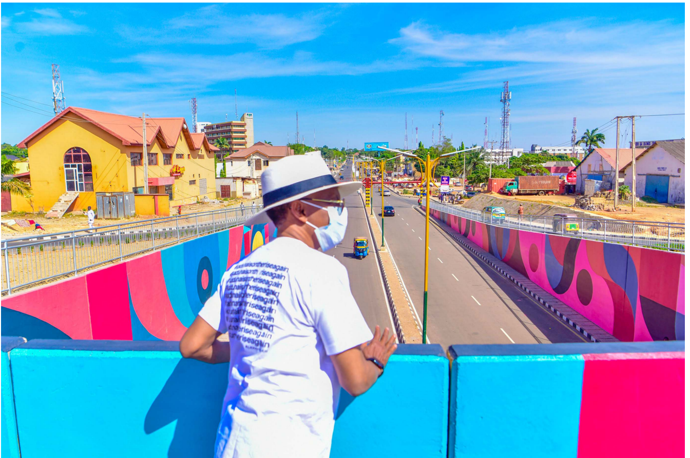
Governor El-Rufai inspecting the newly constructed Leventis Overhead and Under Bridge
