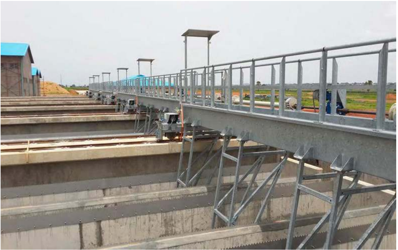
Zaria water treatment plant and Dam
