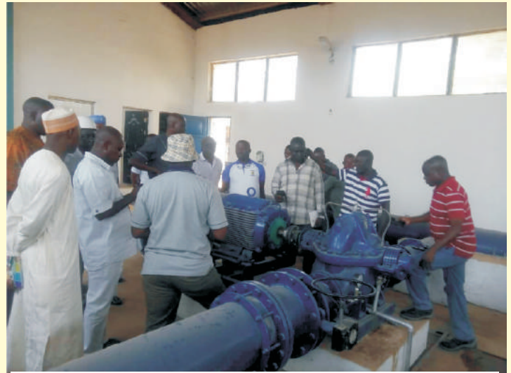
MD, KADSWAC inspecting Booster Stations in Zaria.
