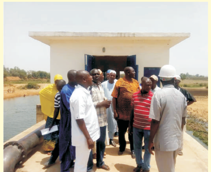
MD, KADSWAC inspecting Zaria Water intake.
