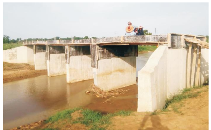
Bridge constructed at River Kiffin by the Shuaibu Goma administration.
