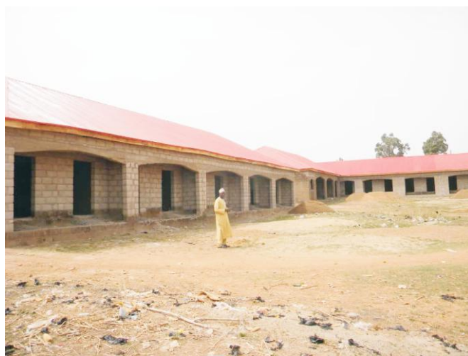
Ongoing construction of Primary School at Ang. Gaye, Kauru LG
